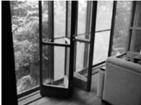
Fig. 6: Window conceived as a folding screen designed by Bruno Taut at Hyuga House. Atami (Japan). (Photo: Jose M Cabeza)
