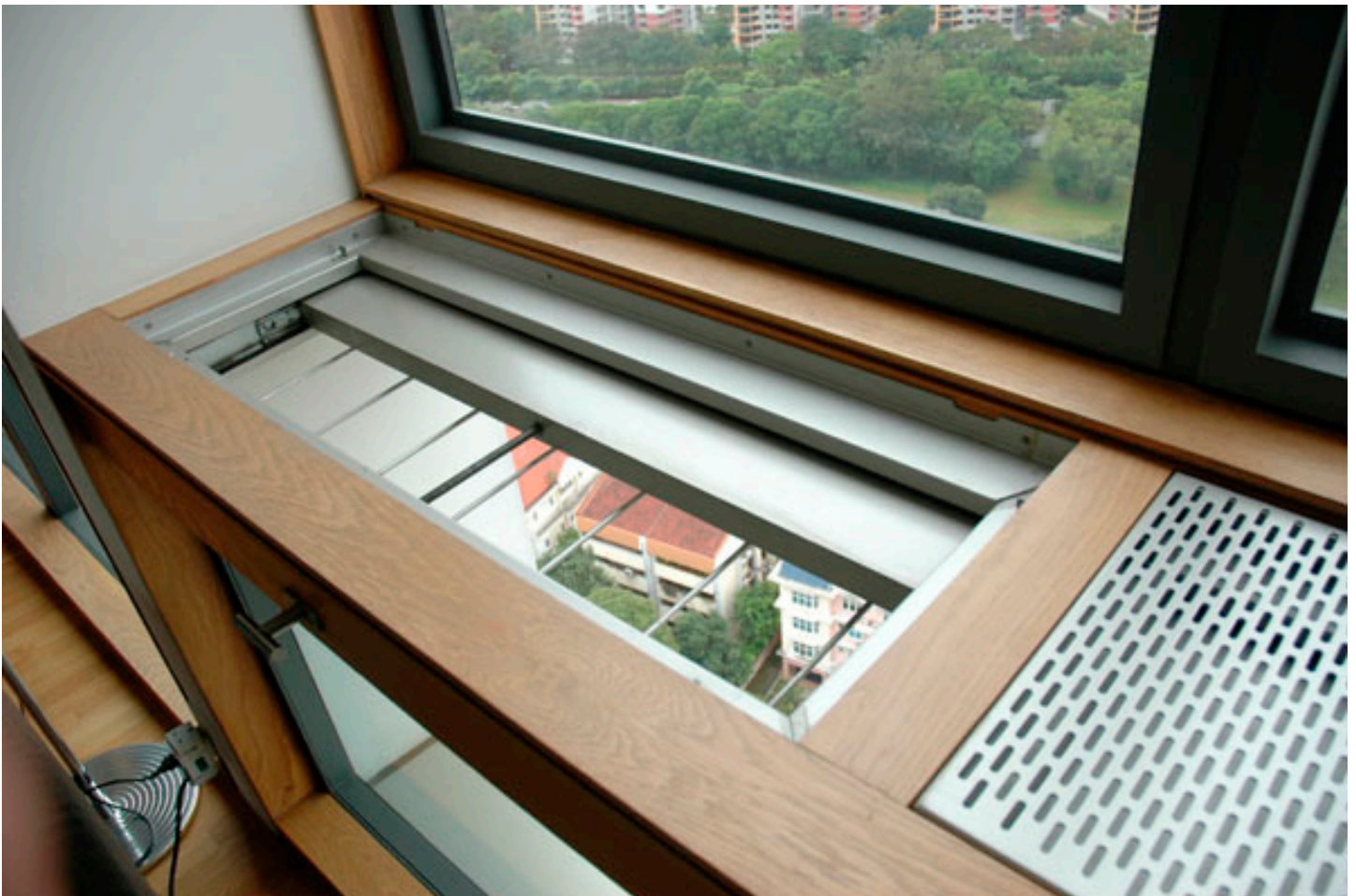
Figure 6: Monsoon window at One Moulmein Rise, Singapore, with slideable panel to regulate airflow. Ventana para el monsoon, con sistema regulable para el flujo de aire.
